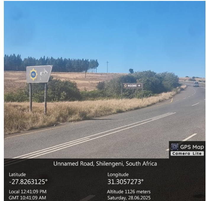
Figure 11-10: Tarred Road with Road Signs
