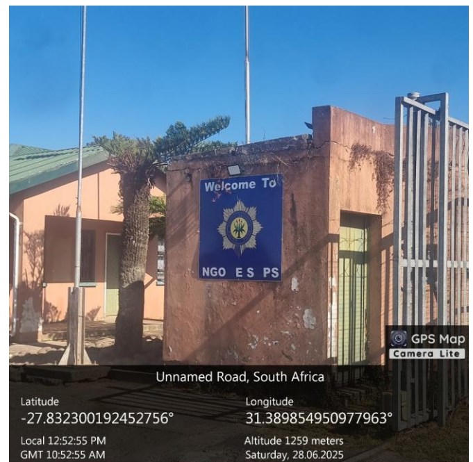
Figure 11-5: Ngome Police Station
